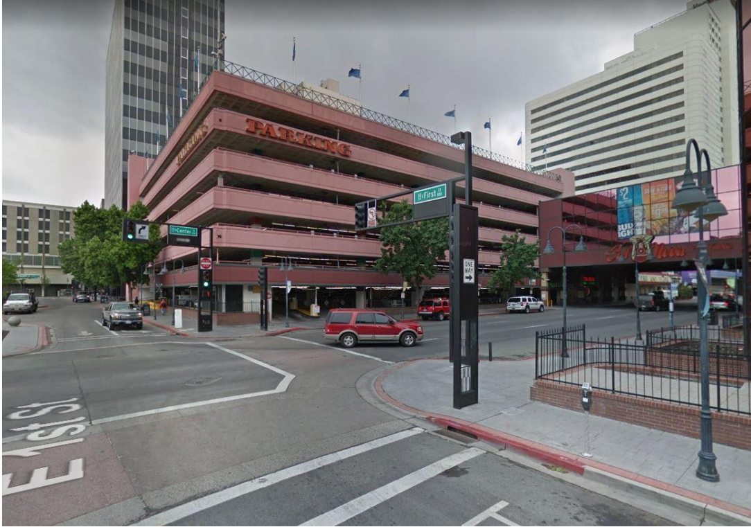
City Hall Parking Structure, southeast corner.
