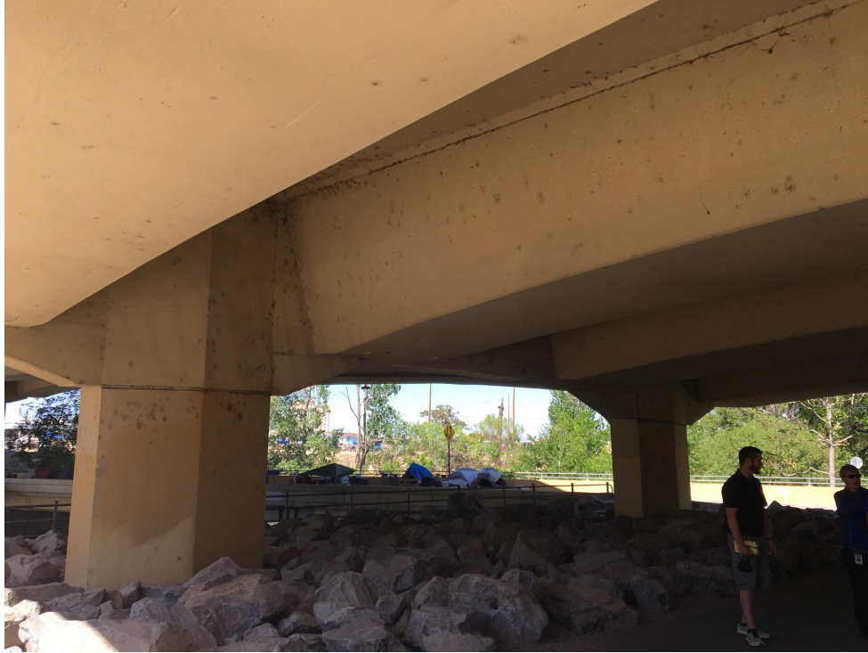
Pedestrian Pathway at Wells Ave Bridge Looking North
