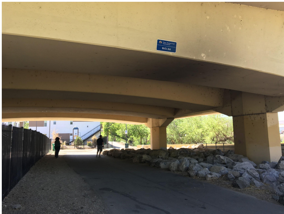
Pedestrian Pathway at Wells Ave Bridge Looking West
