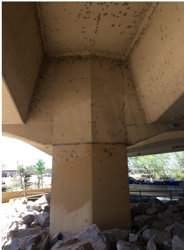
Pedestrian Pathway at Wells Ave Bridge Looking North - Column Detail
