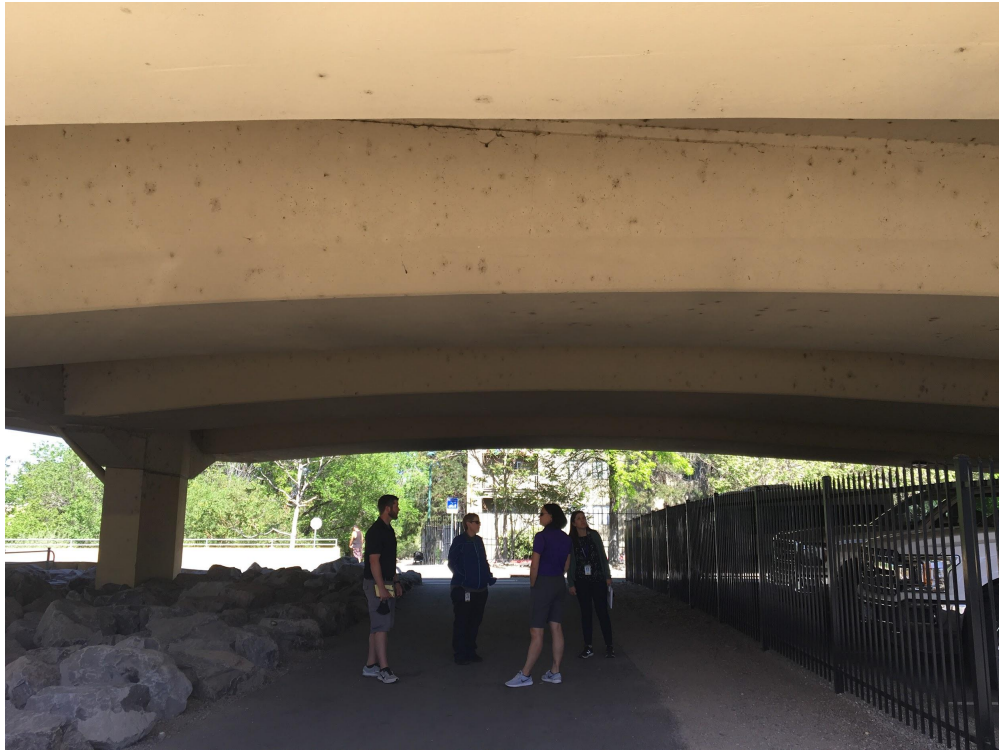
Pedestrian Pathway at Wells Ave Bridge Looking East
